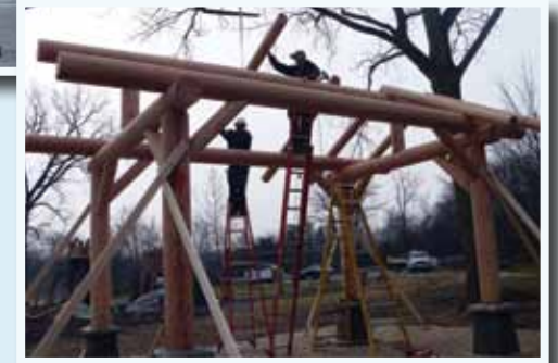
New shelter at Farnsworth
